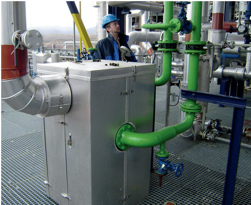
Stainless steel Compablocs were chosen to achieve high quality benzene.
