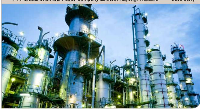
PTT Global Chemical (PTTGC) increased heat recovery in a preheater for a distillation column in one of its aromatics plants by replacing a shell-and-tube heat exchanger with an Alfa Laval Compabloc. The result was 10% lower steam consumption in the column's reboiler and lower maintenance costs. PTTGC is very satisfied with the results and feels confident in using Compabloc for upcoming heat recovery projects.
