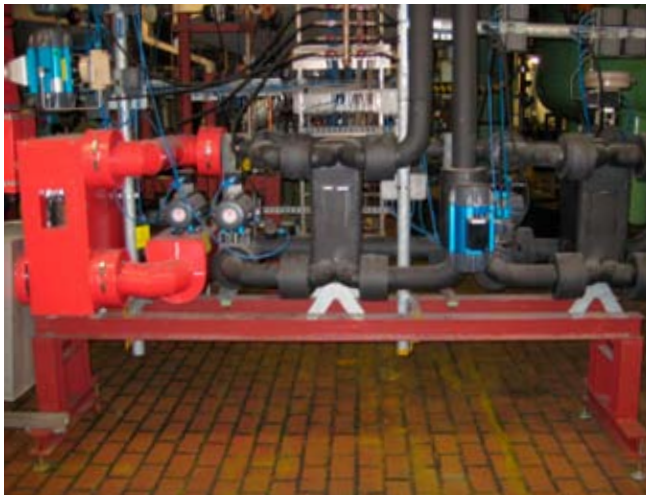
The AlfaNova heat exchangers require minimal installation and piping work, so they are easy to install at the Lanxess plant.
