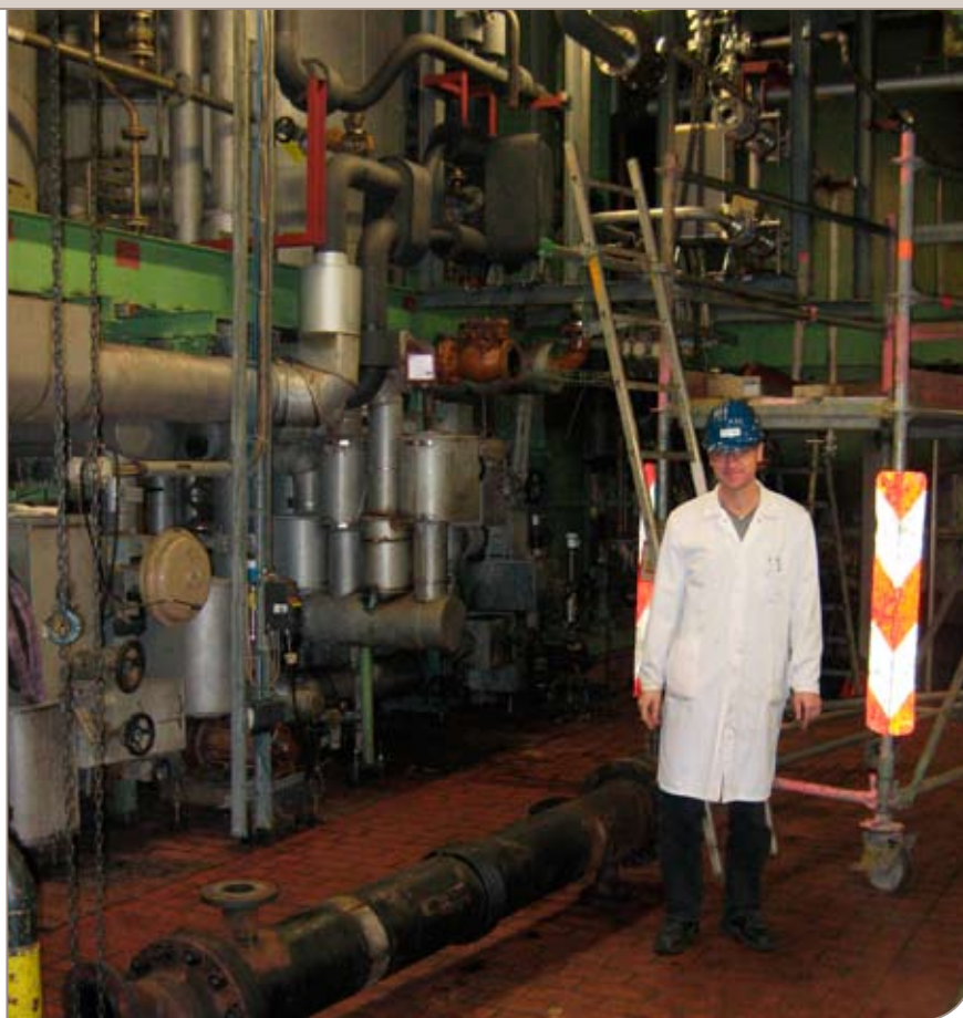
Engineer Holger Kuhr at the Lanxess plant in Leverkusen, Germany standing next to a shell-and-tube heat exchanger that was recently replaced with the compact AlfaNova in the background.
