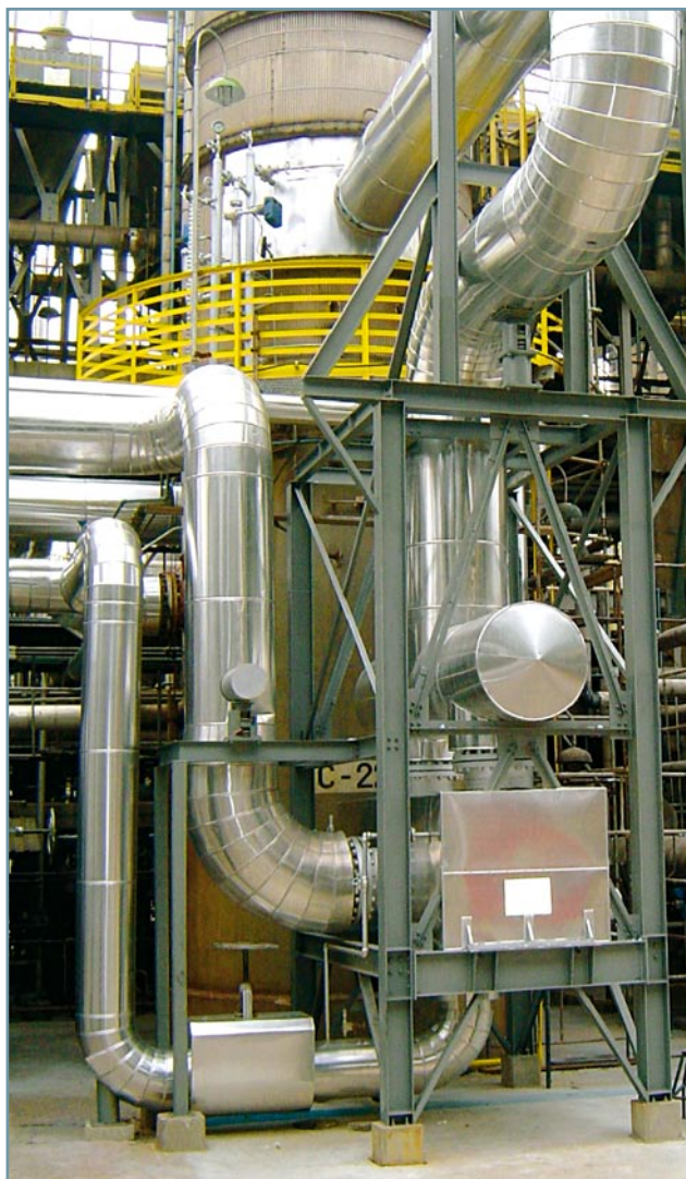
Figure 1. Compabloc reboiler working at the cumene distillation column at UNIPAR in Brazil.
