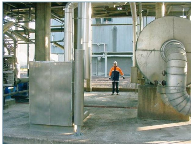
Figure 2. Compabloc working as ammonia cooler at DSM in the Netherlands.
